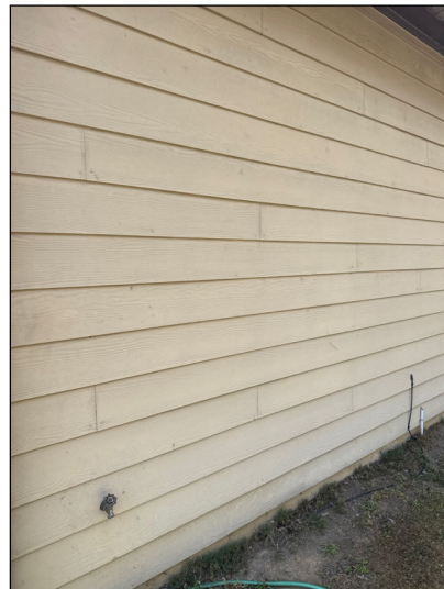
Composite wood siding noted.
