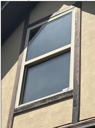
Stucco siding noted
