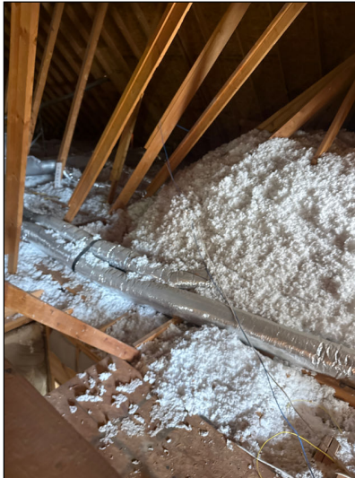
Blown in fiberglass insulation noted.
