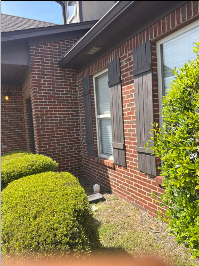
Brick veneer siding noted.
